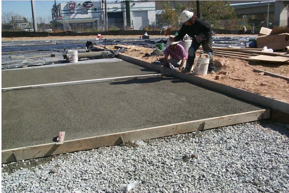
Figure 3-57 Porous Concrete System Installation
