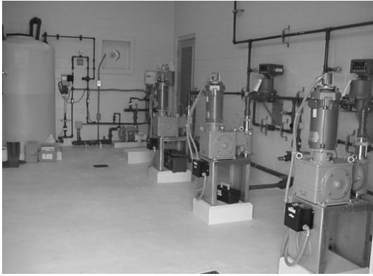
Figure 3-45 Alum Treatment System and Injection Equipment
