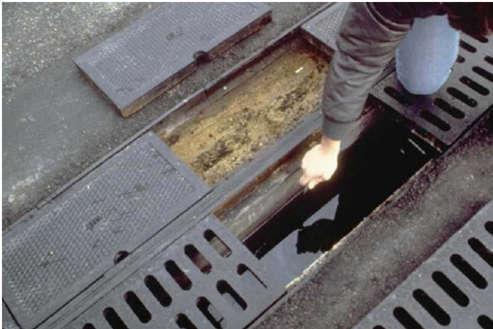
Figure 3-46 Example of an Underground Sand Filter
