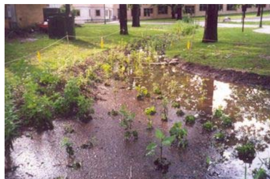
Newly Planted Bioretention Area
