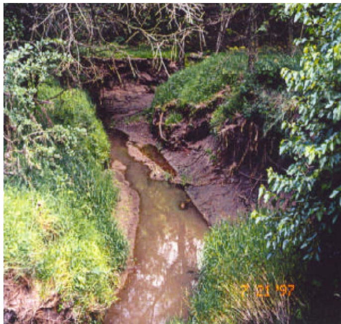
Figure 1-7 Example of Stream Channel Bank Erosion
