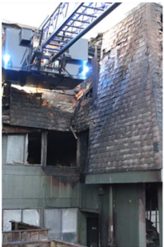
Figure 9: Post-fire damage to the exterior of Building 300. Left: Units 305 (top) 303 (middle) 301 (bottom) and east facing side of exit stairway enclosure. Right: North-facing side of exit stairway enclosure. (Credit: WFD FIU)
